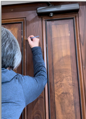
Gail restores the original wood-grained doors
