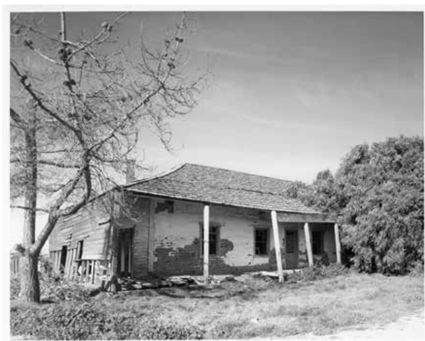
Figure 19. The New Boronda Adobe, main/east elevation, ca 1973.
