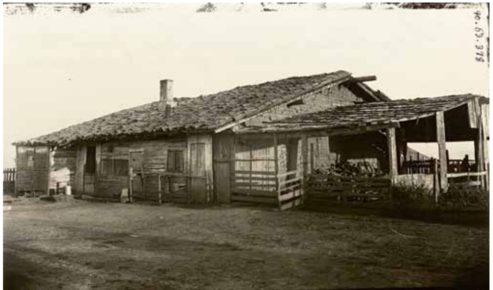
Figure 18. The First Boronda Adobe, rear elevation, ca 1890.
